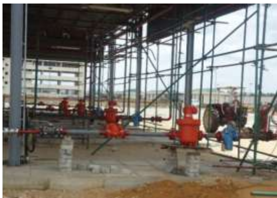
Loading gantry piping and equipment.
