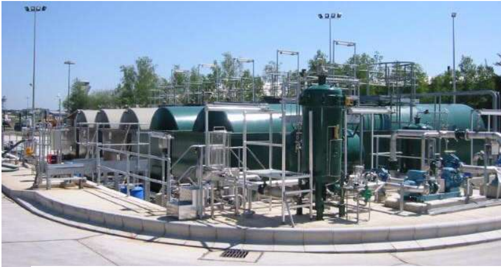
Farnborough Airport, England Design and Build New On Airport Aviation Fuel Tankfarm, Complete June 2003.
