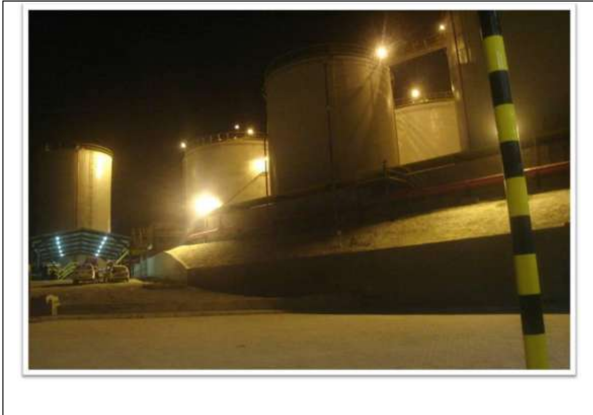
VTTI Kenya, Mombasa Oil Storage Terminal Phase 1 Complete March 2012 - Mechanical & Electrical Design by Trident
