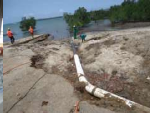
Offshore pipeline connection to the onshore pipeline complete.
