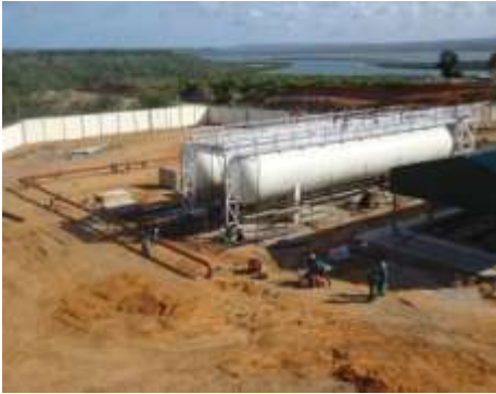
LPG tanks platform and handrails installation in progress.
