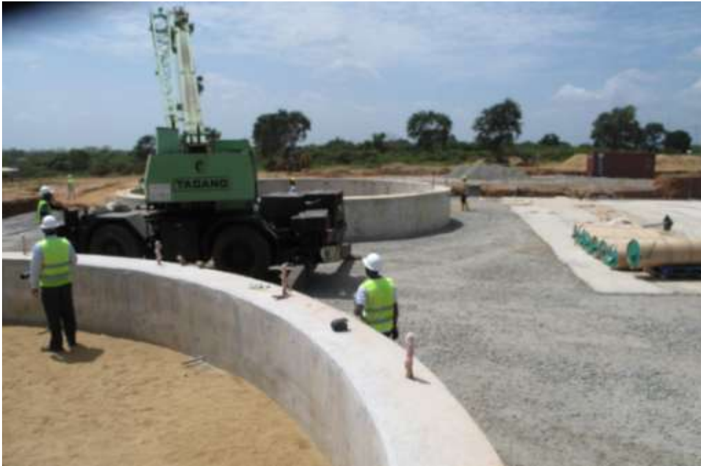
Hambantota Fuel Farm under construction (2012)
