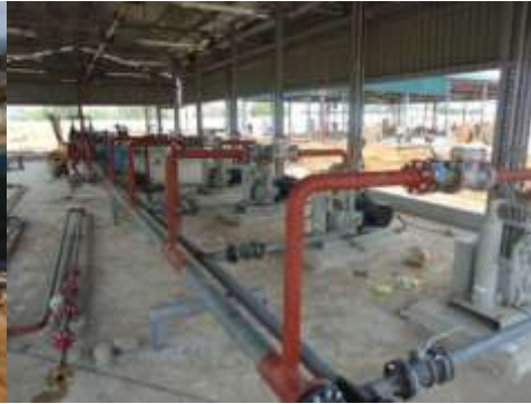
Compressor/ pumps installed and the piping manifold in progress.
