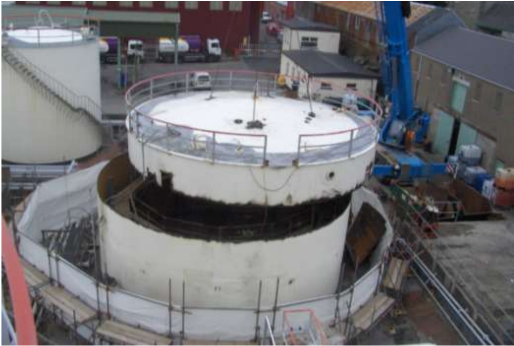
Replacing storage tank (2012)
