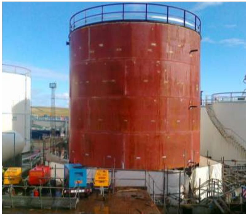
New tank under construction within Lerwick Depot bund
