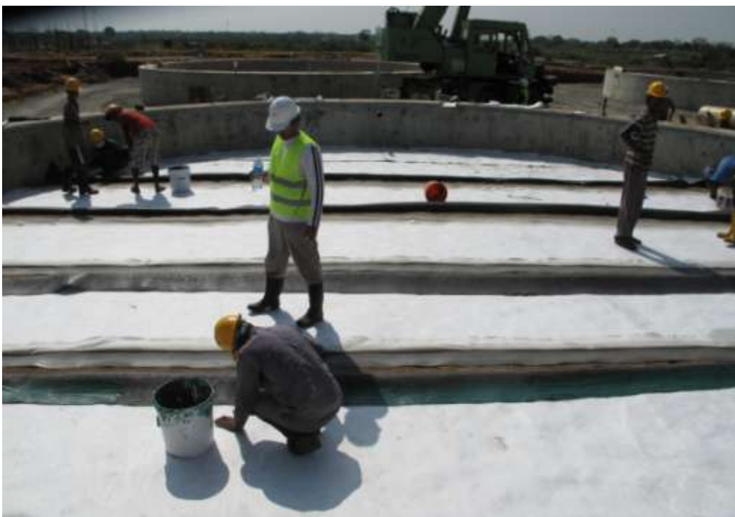
Membrane being installed under new aviation fuel tanks (2012)
